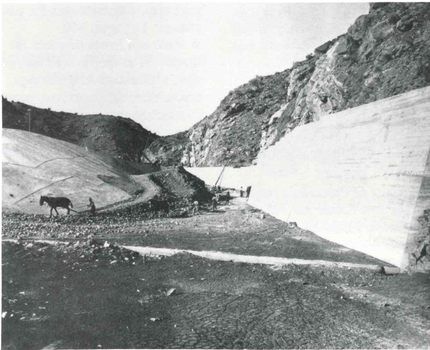
Building the 'Butte - These photos taken during the construction of Elephant Butte Dam (1911-1915) are courtesy of the Rio Grande Historical Collection, New Mexico State University Library.
